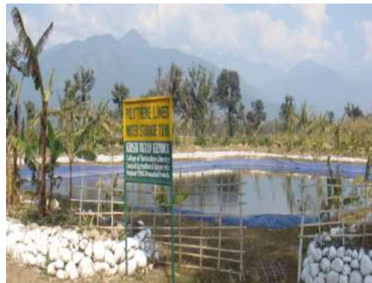
Polythene Lined Water Storage Tank
