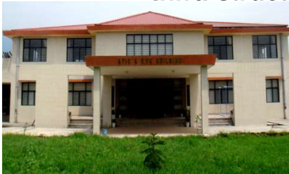
KVK Administrative Building
